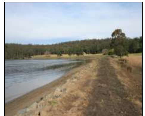
River bank mulched and planted with lomandra, casuarina and a variety of native grasses and shrubs.
