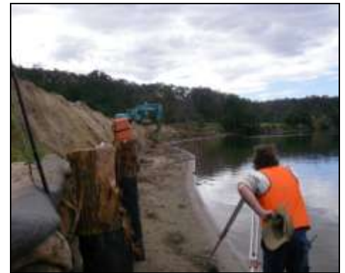
Lyall Bogie, River Rehabilitation Officer (SRCMA) surveying the project site.
