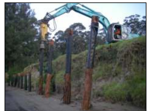
Turpentine log pins being hammered in by an excavator near the boat ramp.
