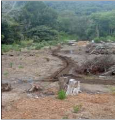
Installing irrigation in preparation for planting
