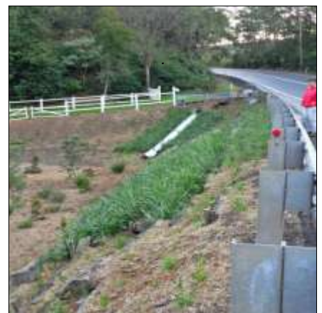
Drain installed and road verge planted heavily with Lomandra cells
