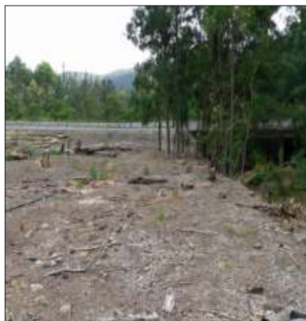
Site after clearing and mulching, with Casuarina stand in background
