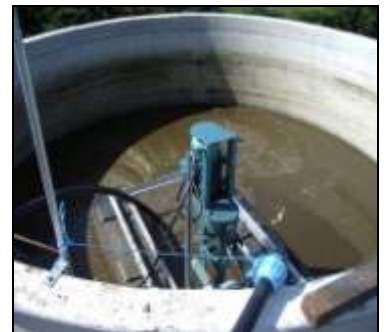
Effluent tank installed below the dairy
