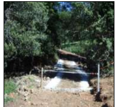
One of five causeways installed.
