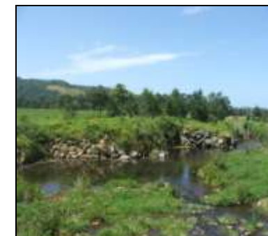
3-yr-old revegetation above 1 of 4 rock structures installed on Fountaindale Creek
